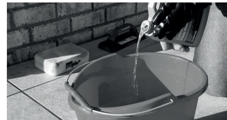
PIC 3. Add specific acid cleaning agent for porcelain tile to clean water.
