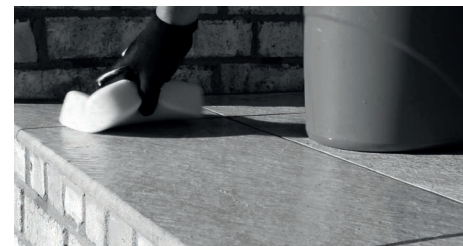
PIC 5. Removal of excess grout residues with hard brush.
