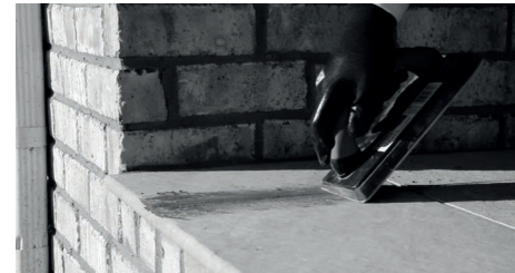
PIC 1. Fill joint with grout.
