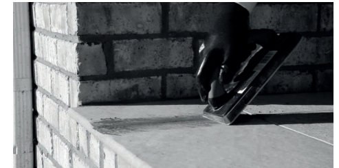
PIC 2. Remove excess grout with clean water.
